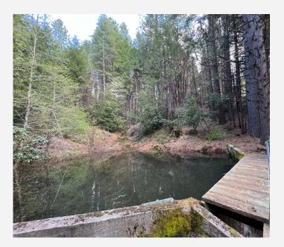
Mill Creek is Foresthill's secondary and/or seasonal water source. This source provides a small but consistent flow of water during winter and spring. Mill Creek is only a seasonal source because it typically dries up in the mid-late summer months. Staff does routine maintenance around the Mill Creek Dam including brush clearing, cleaning, and making minor repairs to extend the life of the structure.
